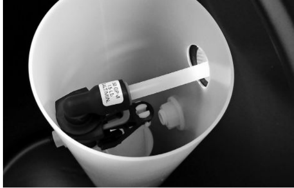
Connection at Brine Safety Float in brine tank
