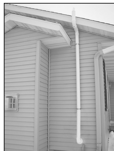
Figure 12 Vent Line Installation (3 inch)
