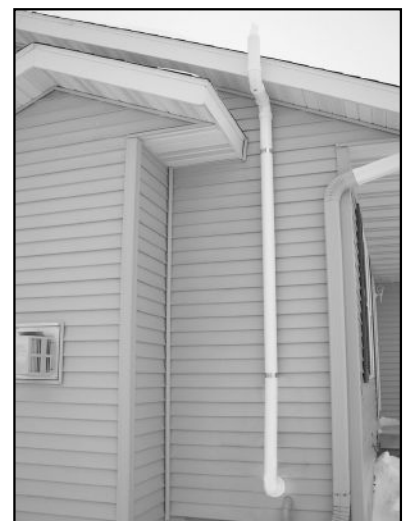
Figure 12 Vent Line Installation (3 inch)
